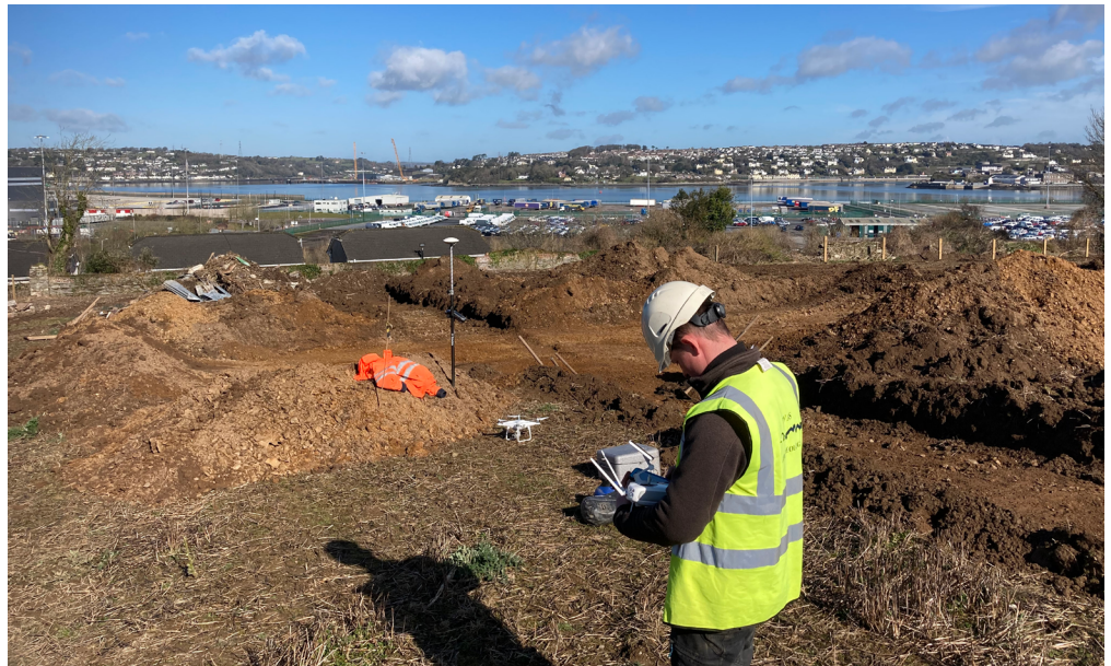
Excavation ongoing in the townland of Loughbeg.
